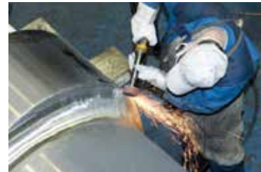
Repair and maintenance measures
